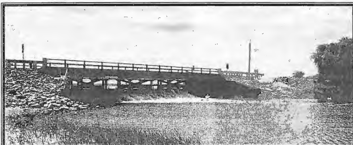
FIGURE D-10 Lake Traverse: Reservation Dam Control Structure
