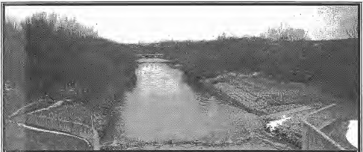
FIGURE D - 18 Lake Orwell: Ottertail River, from Control Structure
