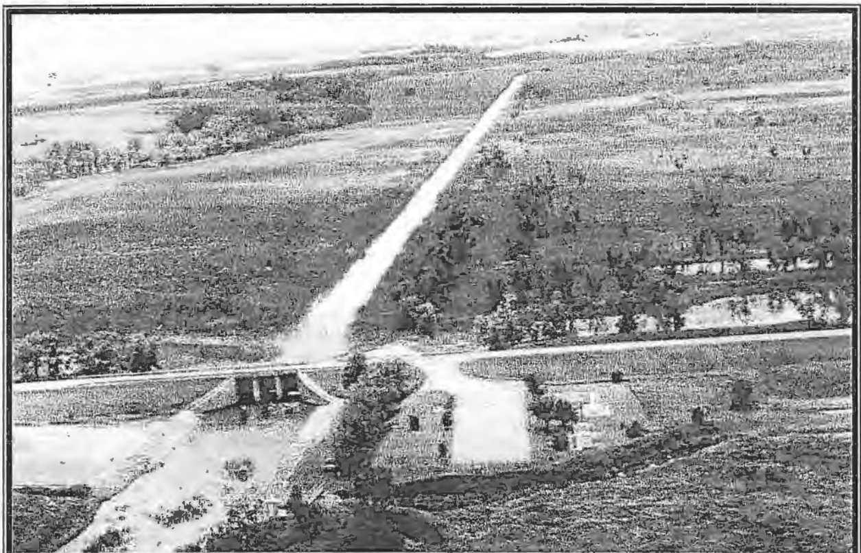
FIGURE 1-8 Lake Traverse: White Rock Dam and Mud Lake
